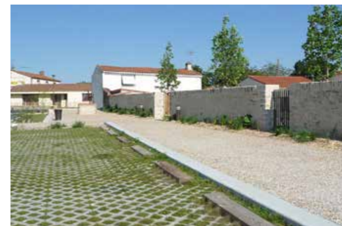
Naturalised green parking reference for Barrack Street (Zephyr-paysages, Place de Chevigné – Saint-Fulgent, France)
